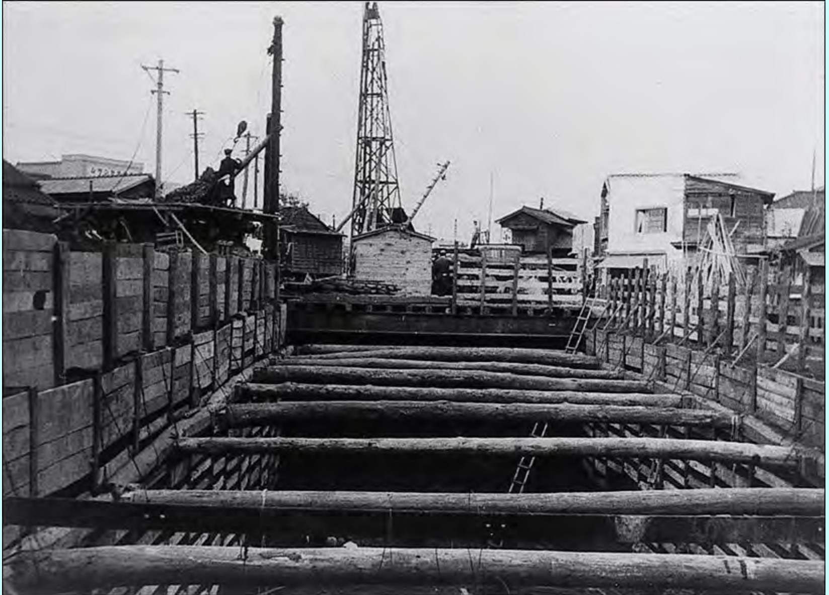
Pine log Wooden support (Marunouchi line)
