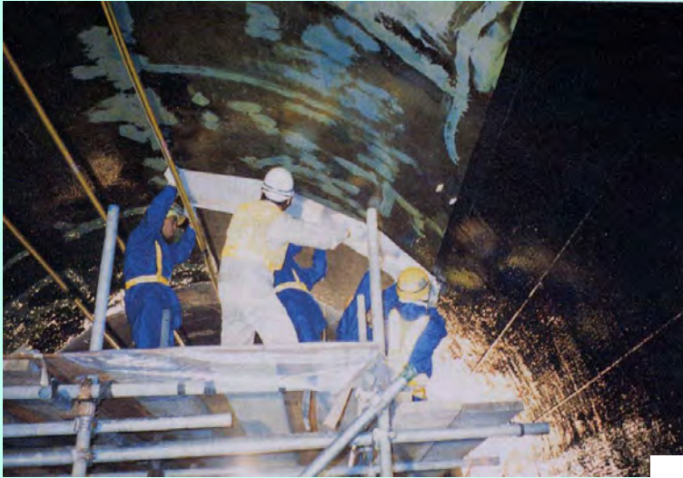
An example: an application of carbon fiber sheet lining method
