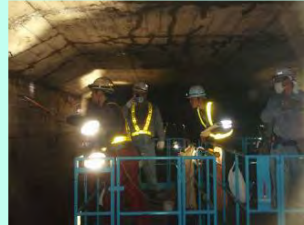
Observation from near, Hammering
