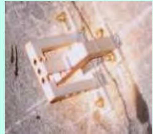
Crack width measurement
