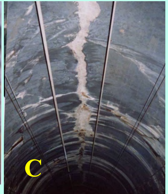
Compressive failure
