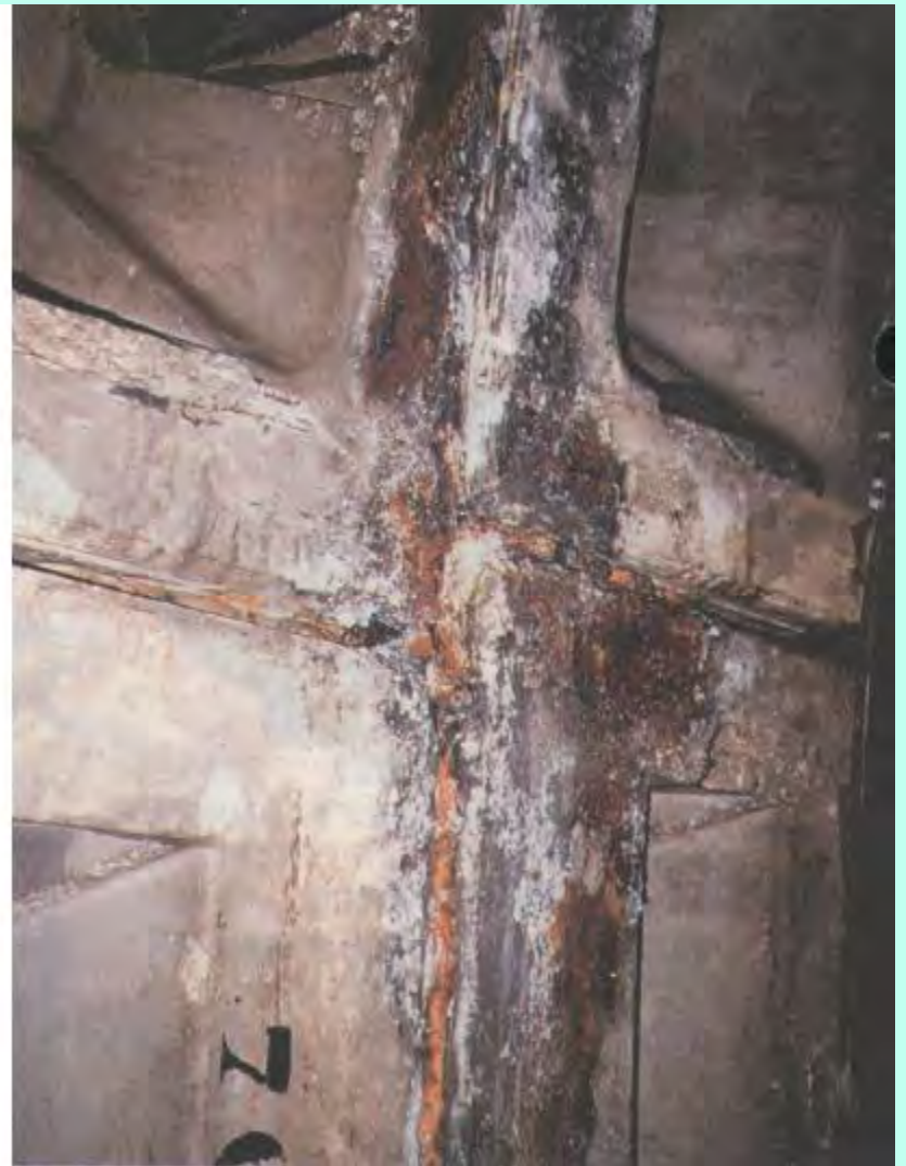
Degradation of segments and joints
