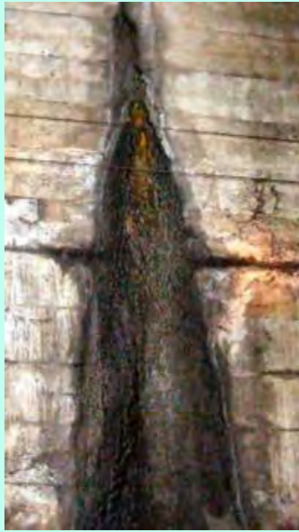
Inner tunnel surface
