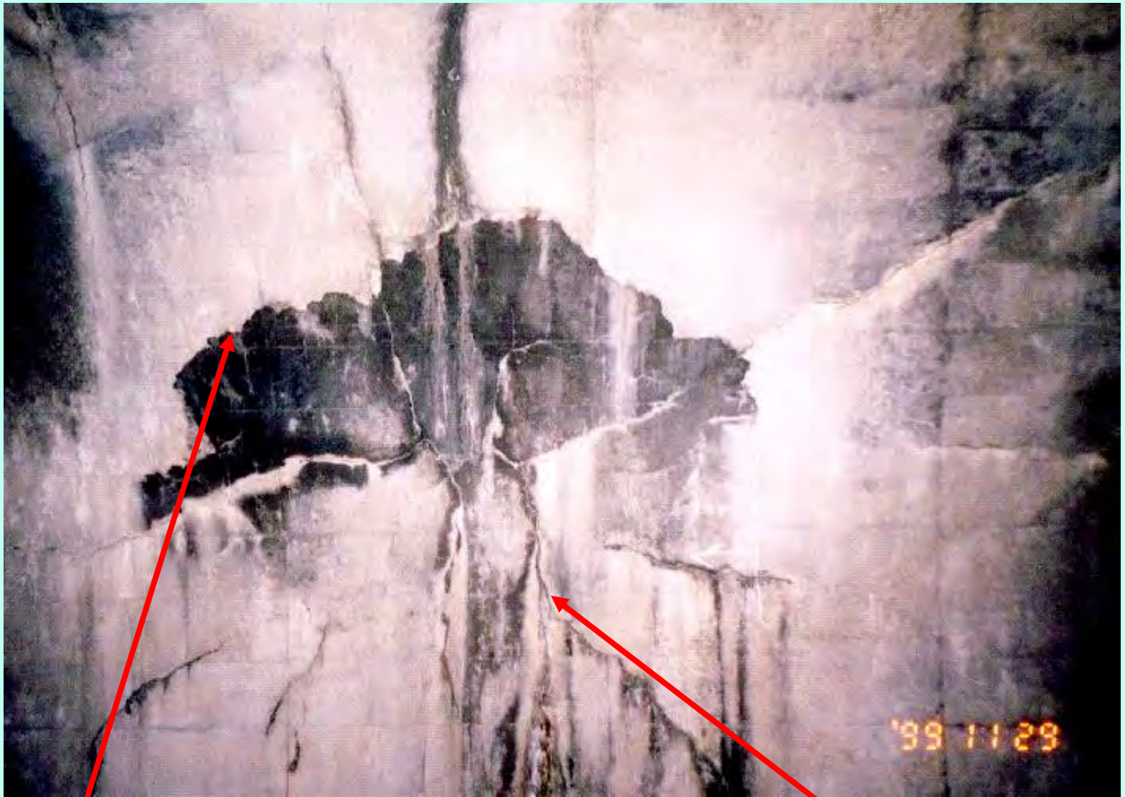
Radial cracks
