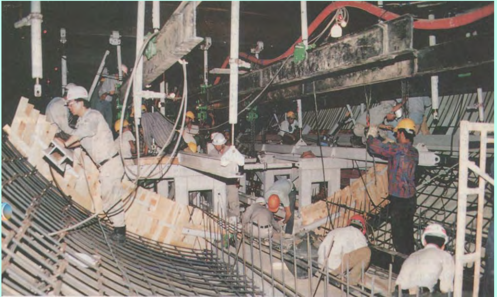
Assembling reinforcing bars of the secondary lining
