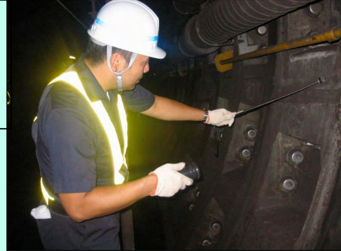
Hammering on lateral of segmental lining
