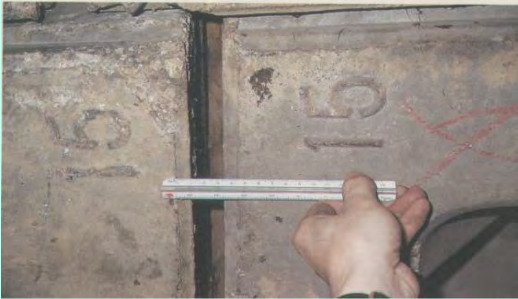
Aperture of a joint
