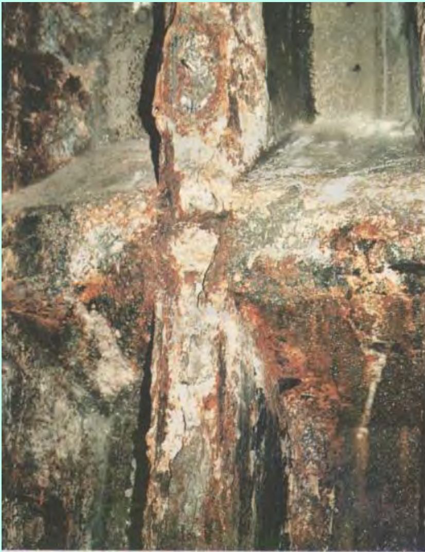
Degradation of segments and joints
