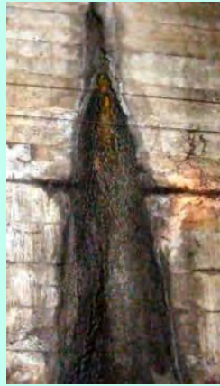
Inner tunnel surface
